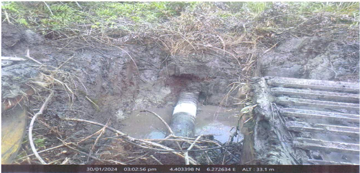
Repaired incident point
