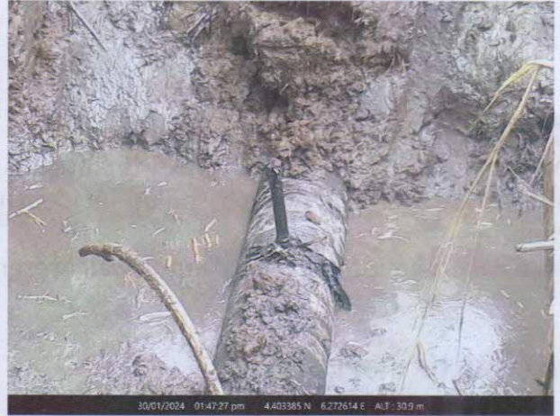
Incident point with 2" Valve with pipe Connection Installed.
