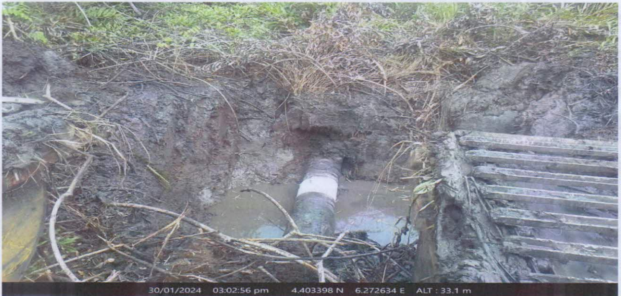
Repaired incident point
